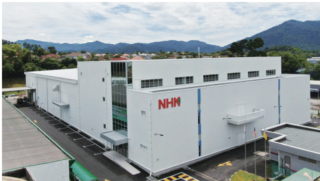
NHK NEW FACTORY PROJECT
